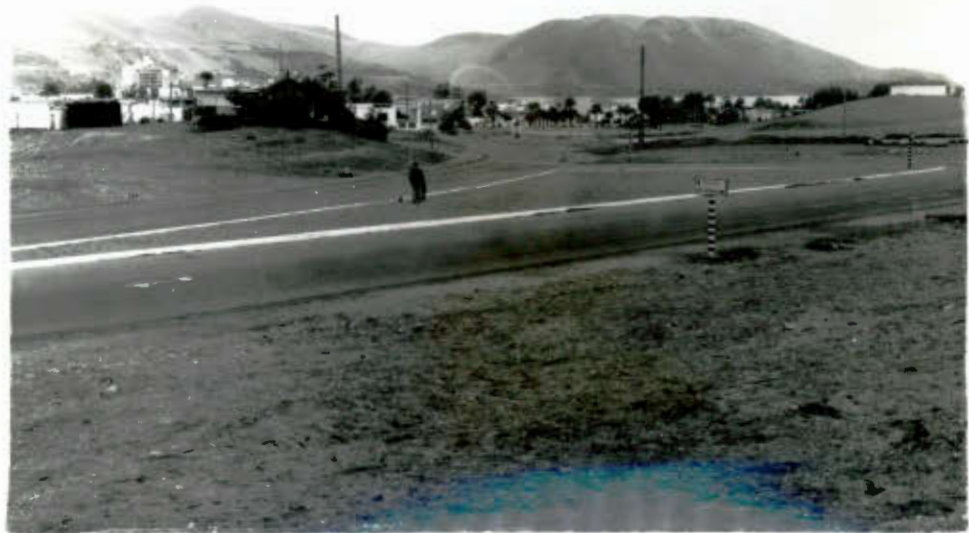
Carretera Lima-Ancón Km, 35
