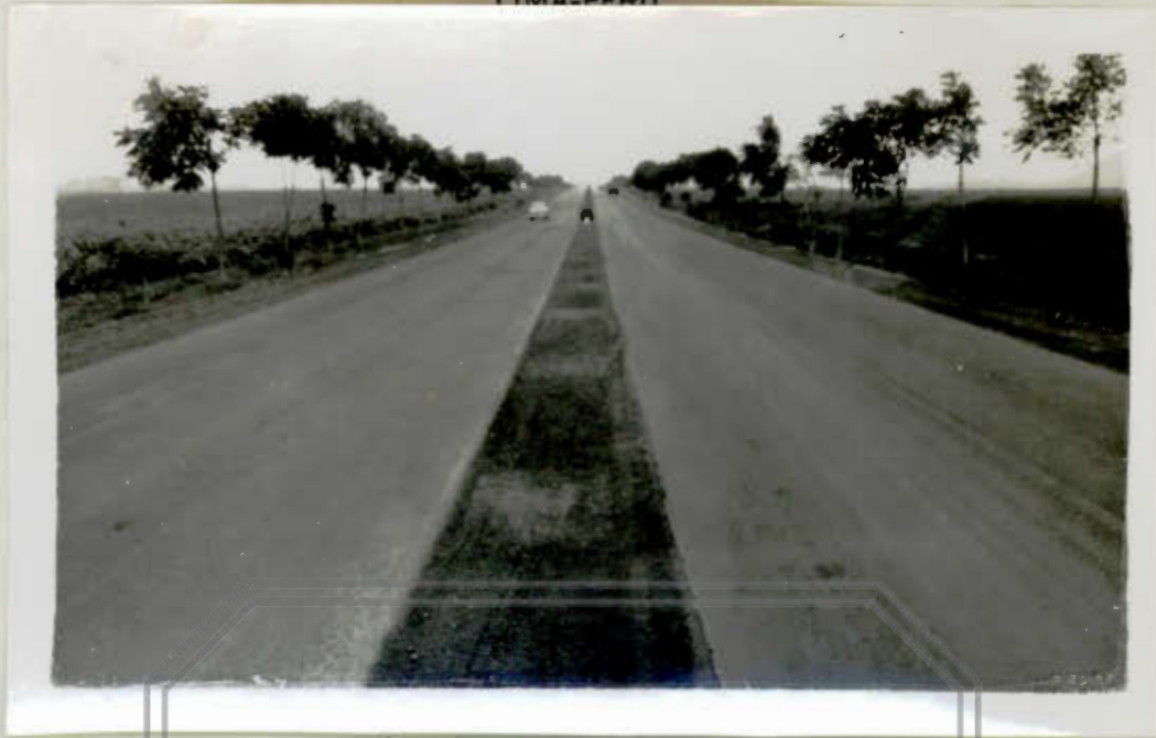
Carretera Lima-Ancón Km. 5
