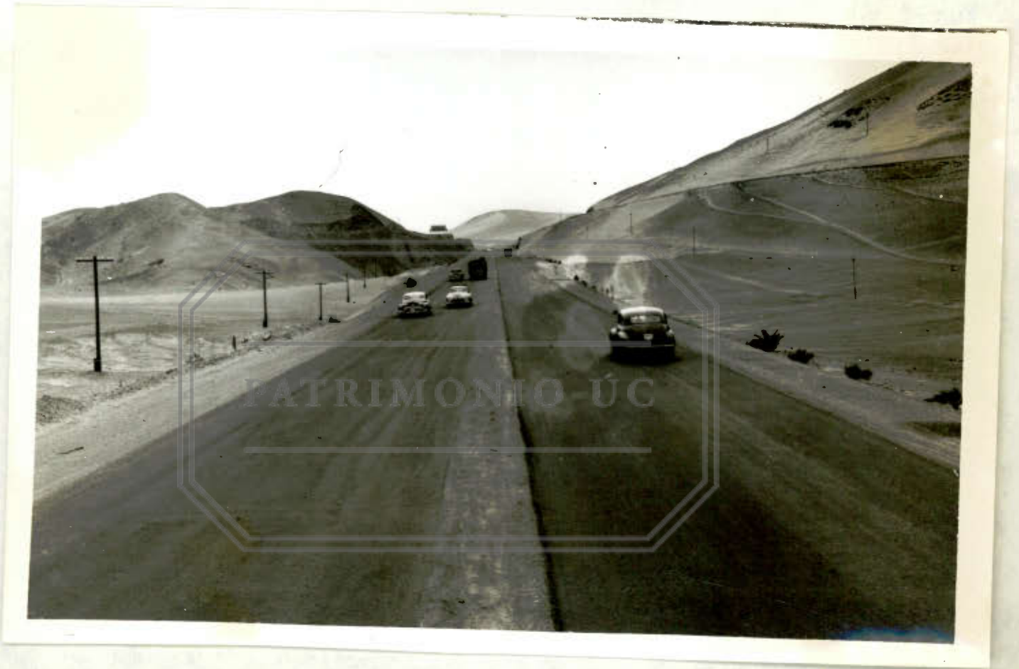
Carretera Lima-Ancón Km. 30
