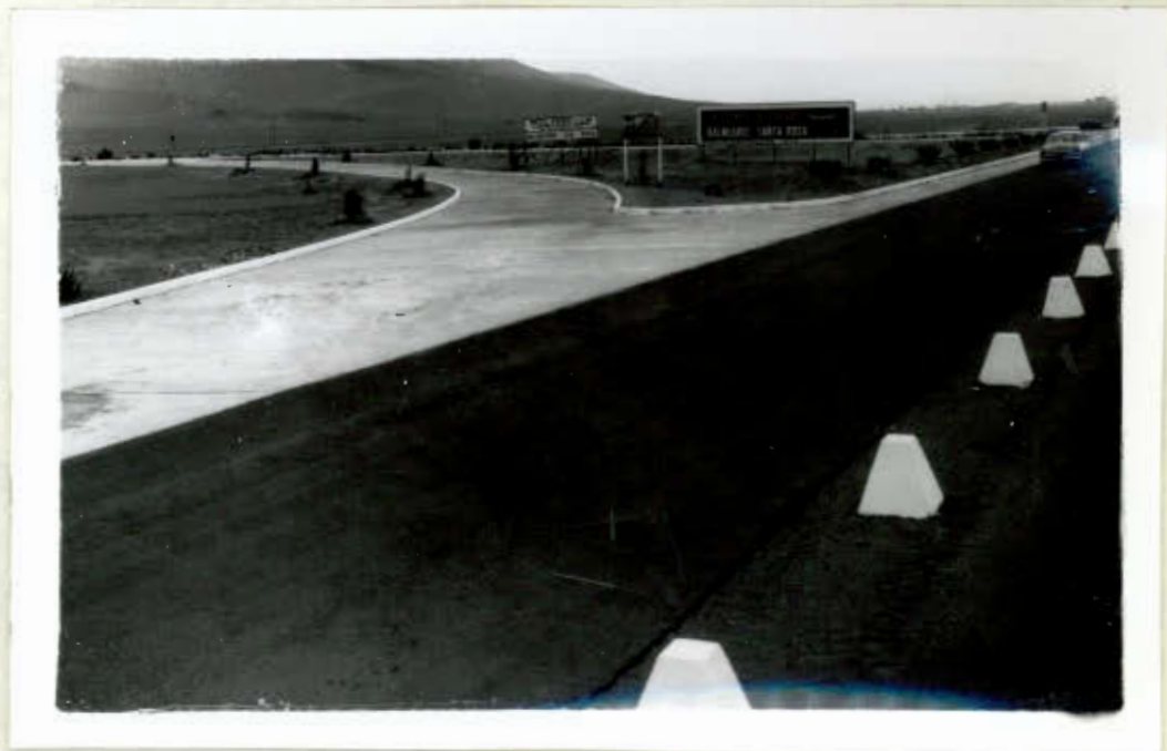
Carretera Lima-Ancón Km. 32
