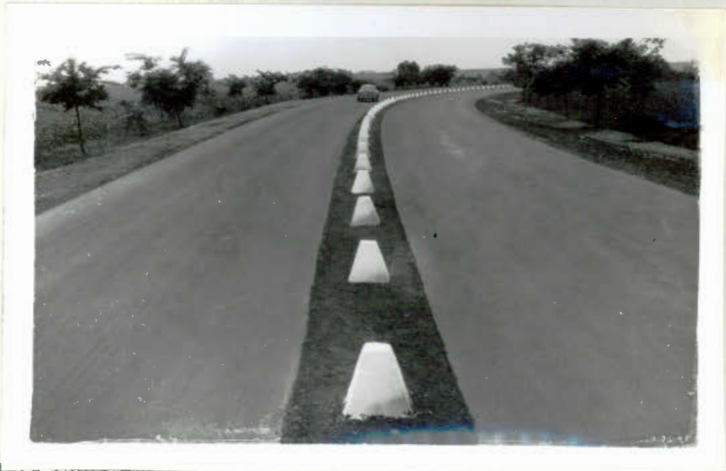
Carretera Lima-Ancón Km. 16
