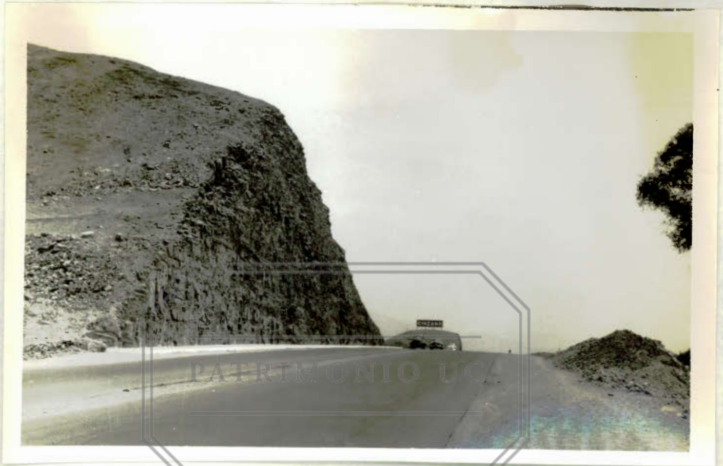
Carretera Lima-Ancón Km. 16
