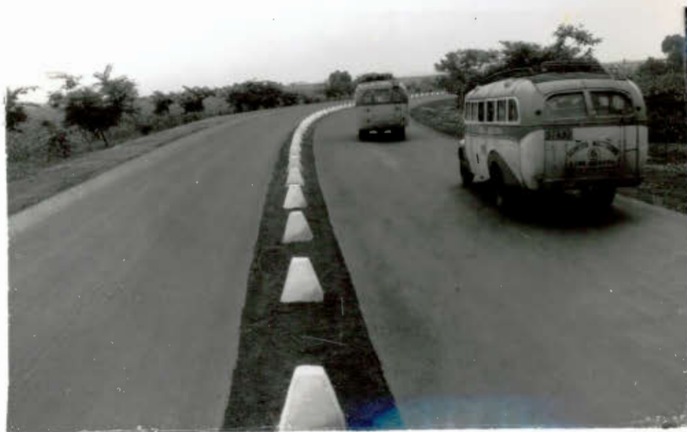
Carretera Lima-Ancón Km. 16
